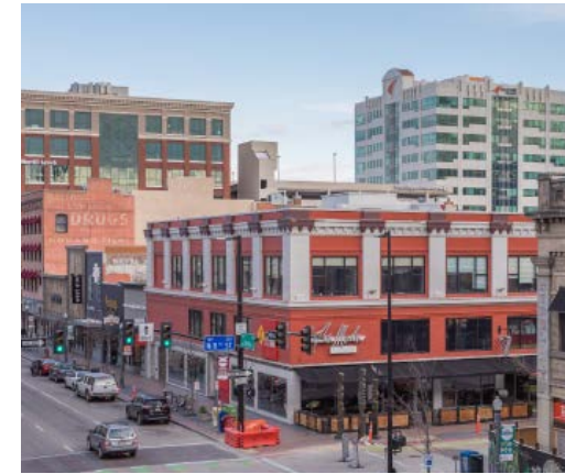
URBAN REDEVELOPMENT Two City Blocks Downtown Boise 44,202 SF | Boise MSA
