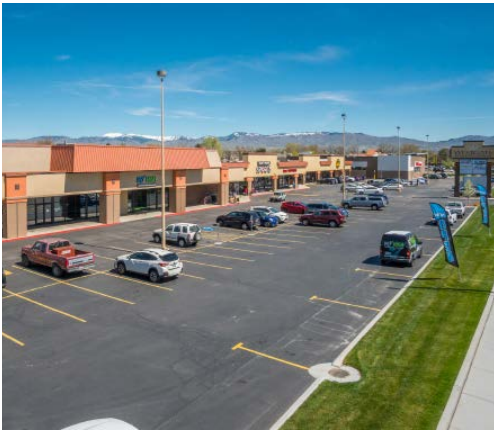
RETAIL CENTER REMODEL CVS Build-out 61,512 SF | Boise MSA
